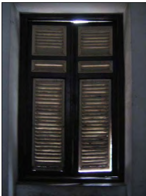
Figure 10 the picture showing the window that deteriorated by humidity and micro-organism.
