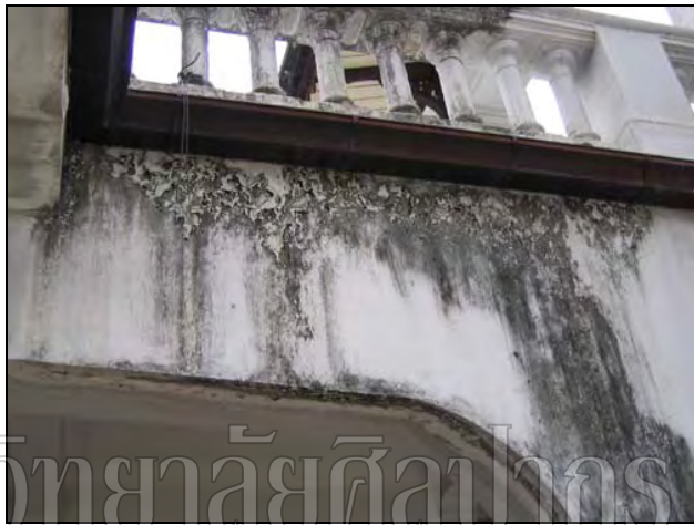
Figure 11 the picture shows the stucco deteriorated by humidity and microorganism, caused by gutter malfunction.
