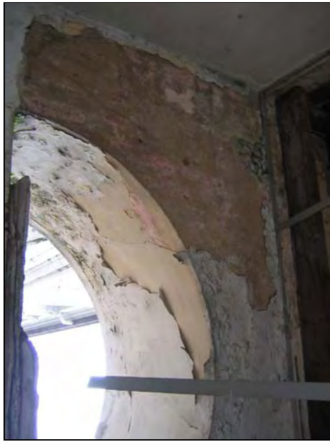
Figure 15 the picture showing the result of deterioration by painting application on mortar.
