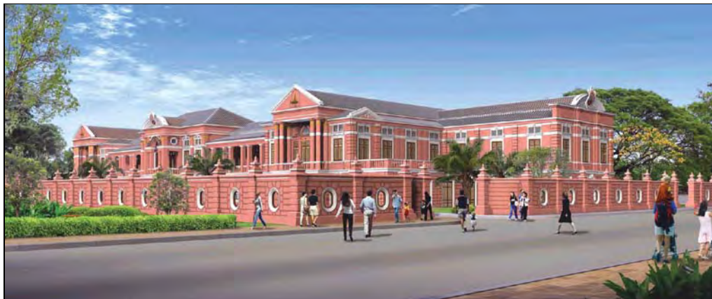
Figure 16 the perspective picture showing Saranrom Palace after the conservation process.
