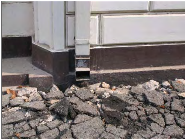
Figure 19 the picture showing the drainage around the building which is obstructed by debris.
