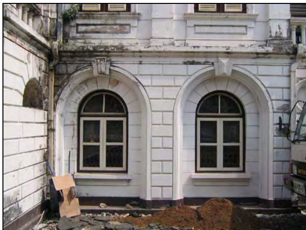
Figure 12 the picture shows the stucco deteriorated by humidity and microorganism, caused by the leakage of downspout.
