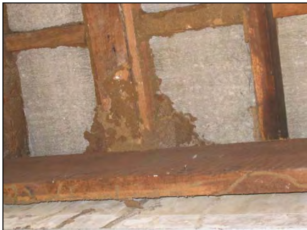
Figure 16 the picture showing the deterioration by termite attack.
