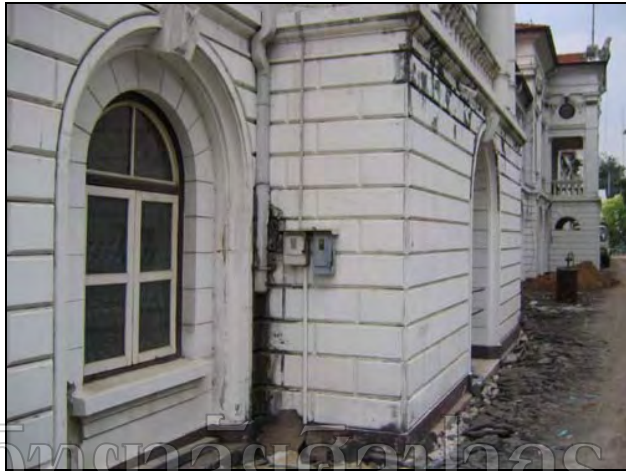
Figure 17 the picture showing the malfunction of the downspout.
