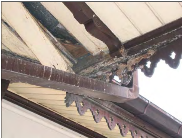
Figure 8 the picture showing the deteriorated roof.
