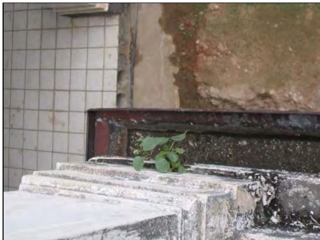
Figure 18 the picture showing vegetations threaten the gutter.
