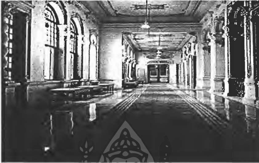
Figure 22. Verandah on the upper floor
