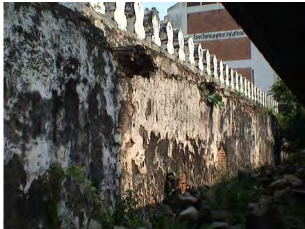
Figure 9 Palace Wall inside
