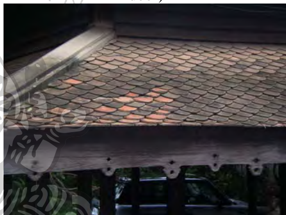
Figure 17 Ginger Bread on the roof decoration of the Wooden Pavilion and discoloration on the roof tile
