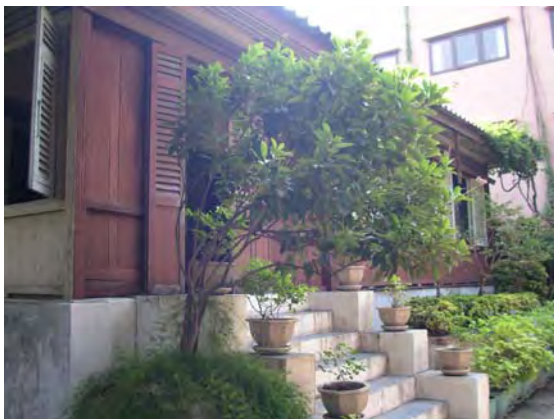
Figure 62 West side (front) of the Residential Building
