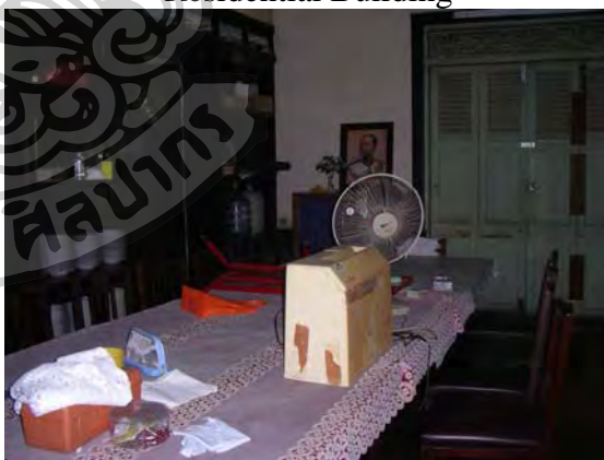
Figure 43 Close door and discoloration of the first room
