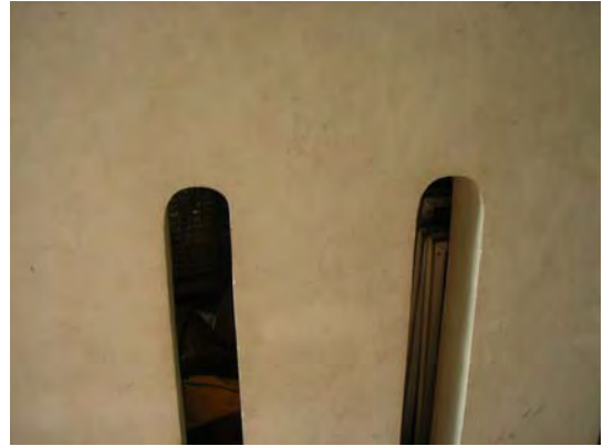
Figure 33 Ventilation vent on the rising platform
