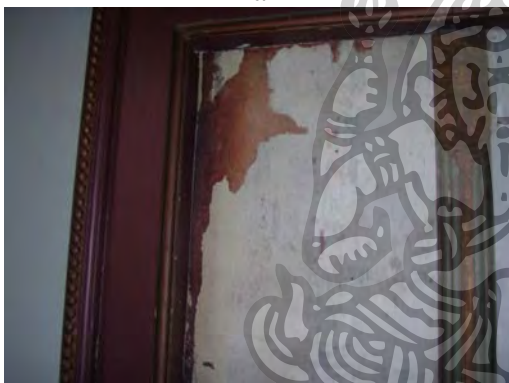
Figure 10 Peeling color cause by human
