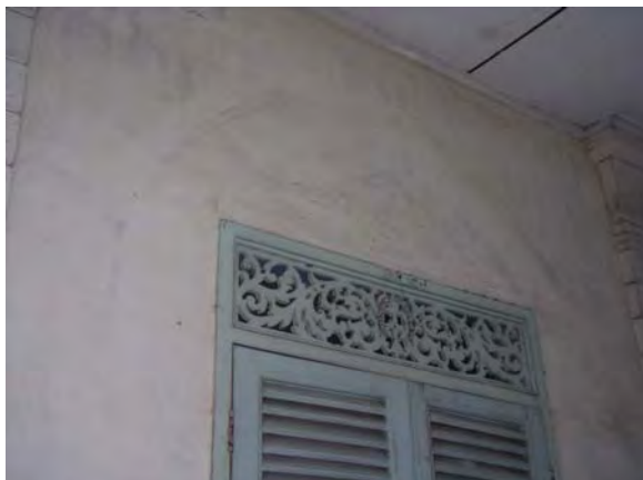
Figure 56 Evidence of arch above the window decoration
