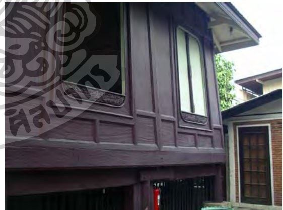
Figure 31 Fire extinguisher hanging on the Audience Hall
