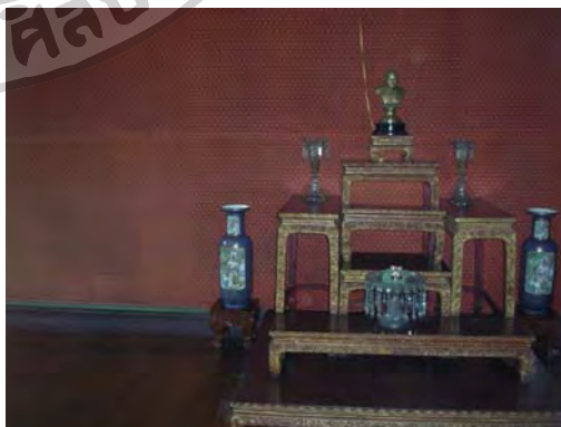
Figure 13 Discoloration on the partition of the Main Hall
