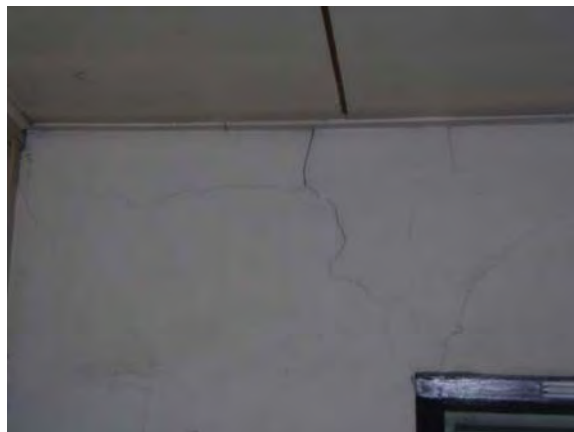
Figure 45 Different settlement on the wall
