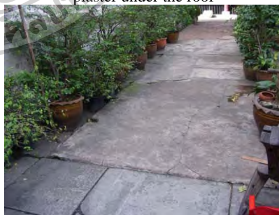
Figure 73 Contrast between an old pavement and the new concrete pavement
