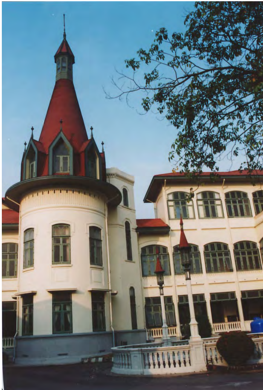
Figure 109 Street lights form is as same as roof form
