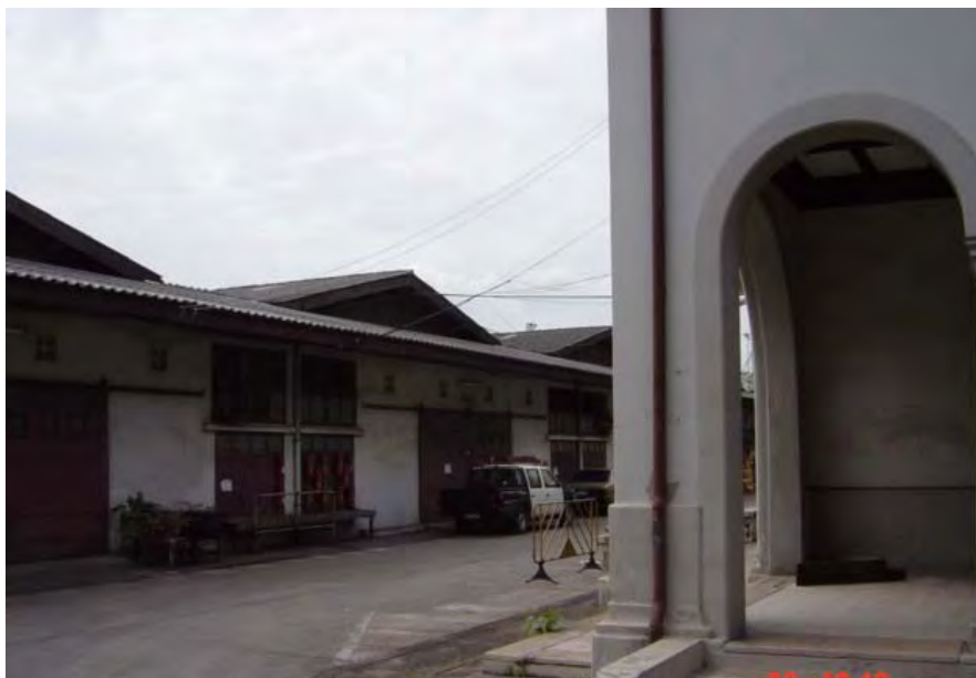
Figure 9 South, In front of Police Quartermaster Depot
