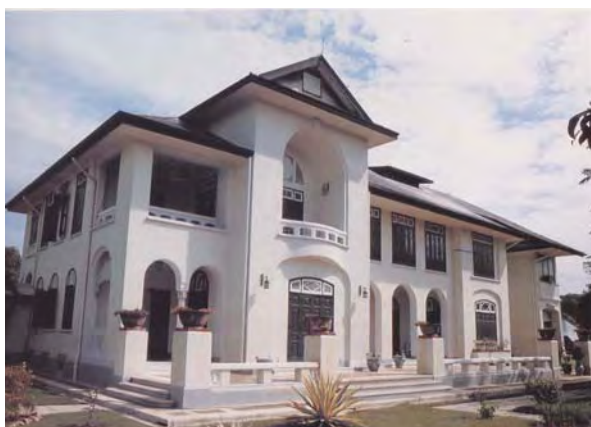
Figure 17 Somdej Jaofah Kromluang Songklanakarin mansion, the example of house in the reign of King Rama the Seventh.
