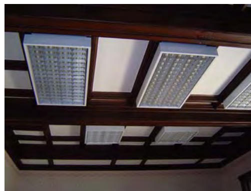
Figure 46 While the fluorescent lamps should be changed to serve the purpose of the museum and conservation.
