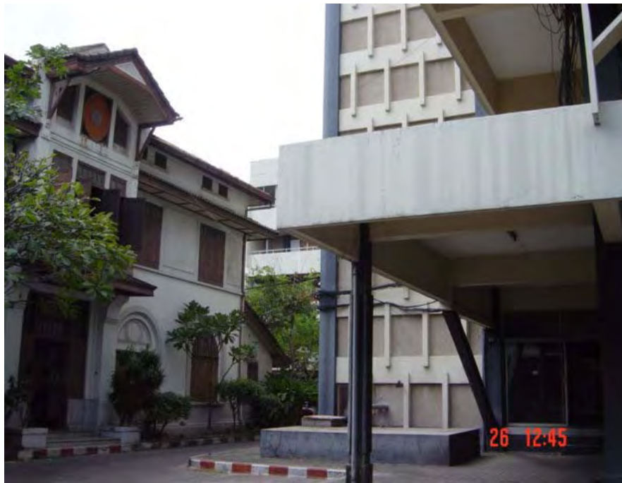
Figure 8 North, Behind Police Quartermaster Office Building
