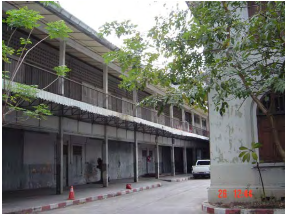
Figure 10 East, Close to Office Parking lot
