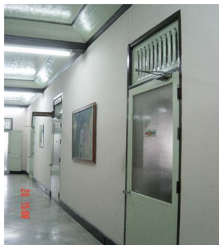
The old wall and doors
