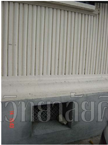
View of front elevation. Damage of wall and window-sill, Window-sills in the pictures seriously damaged, its color scratched and peeled to show lime mortar inside.
