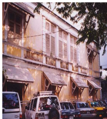
View of Northwestern corner and west elevation of the building. Deteriorated fabric clearly seen, especially on the wall of closed terrace where there is no sunshade.
