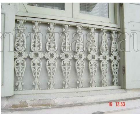
Figure 108 Beautiful metal curved railing is in a good condition but wall plaster moulding and wooden frames of window are in bad damage of color peeling and scratch.
