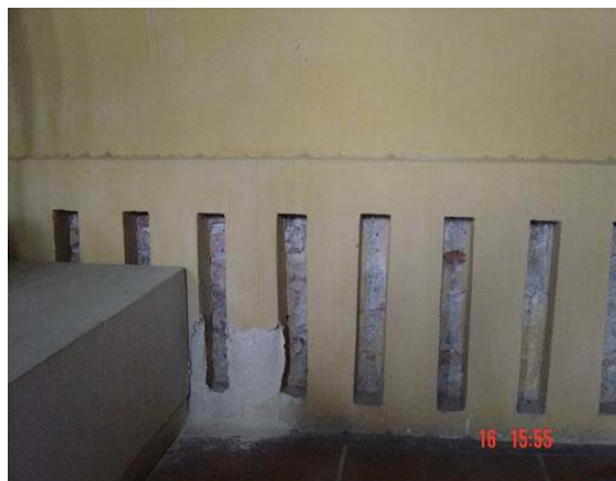
Wall painting is scratching and peeling. The serious problem is lime stucco corrosion.
