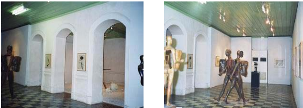
Figure 57 View of room no.3. The original decoration and materials remain such as arch void, marble floor and old style clay tiles border. Some parts of wall were attached with gypsum board wall. Electrical lights and facilities were installed. There are some cracks on the wall.
