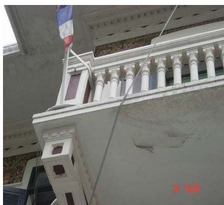
View of front elevation. Under the balcony and sunshade has deterioration of cement stucco caused by rain and may be water leaking on the top of sunshade.
