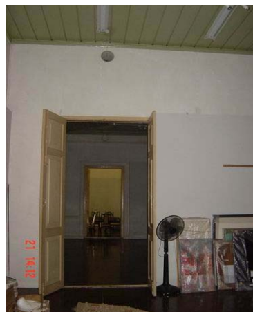
View through the room from north to south
