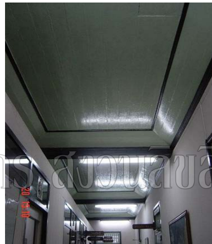
Ceiling over corridor
