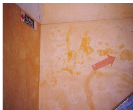
Staircase wall, view from ground floor. Condition of wall painted is bad. Discolor and color patches are clearly seen. Design of direction signs is out of date and uninterested.
