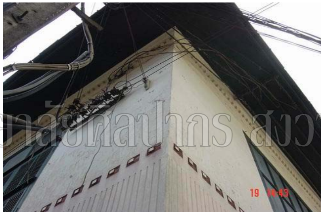
Disorder of electrical wires, it is not only affecting to the beauty of building but also causing of hazardous.
