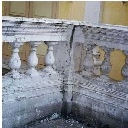
The balcony has bad condition of color scratch and peel. It dirties with fungus stains and waste from birds.
