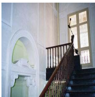
Stair case and walldcoration, view down from upstairs.
