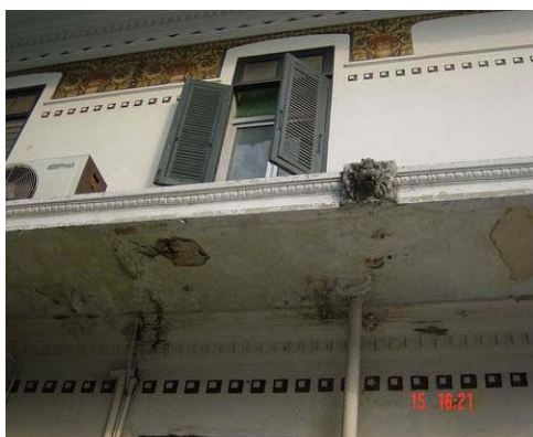
Back of the building show serious damages of wall and sunshade. Some significant decoration lost.
