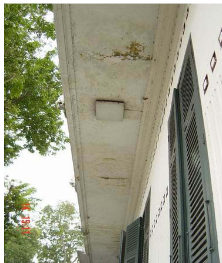
View of front elevation. Under the balcony and sunshade has deterioration of cement stucco caused by rain and may be water leaking on the top of sunshade.
