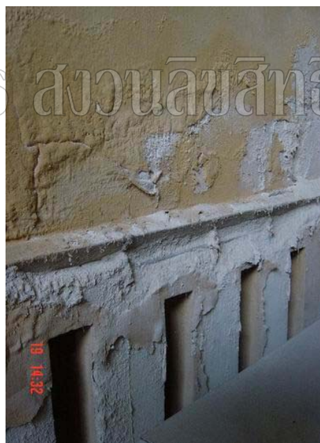
Wall painting is scratching and peeling. The serious problem is lime stucco corrosion.
