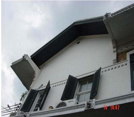
North side of the building has different form of roof and upper sunshade from the south side.
