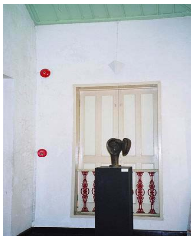
West elevation, having decorated light and fire alarms.
