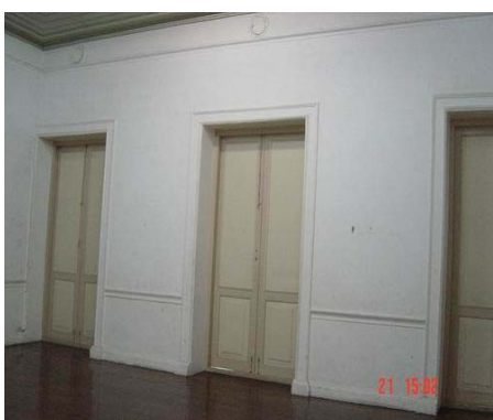
Front wall of middle room ( Room no.5 ).
