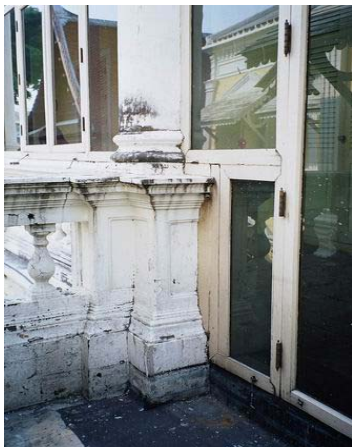
The balcony has bad condition of color scratch and peel. It dirties with fungus stains and waste from birds.
