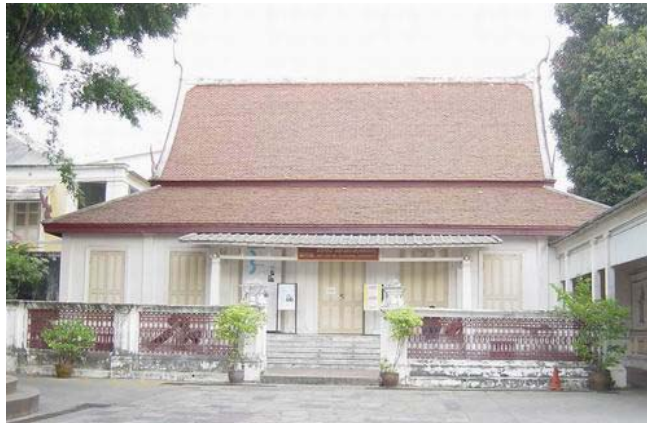
Figure 35 Front elevation of Thong Phra Rong in Wang Tha Phra see from the main gate.
