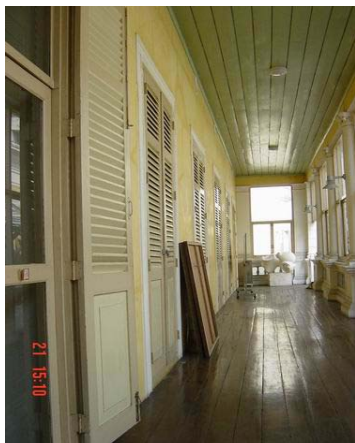
Terrace view from staircase. Overall condition is satisfactory.
