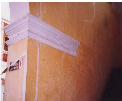
Staircase wall, view from ground floor. Condition of wall painted is bad. Discolor and color patches are clearly seen. Design of direction signs is out of date and uninterested.
