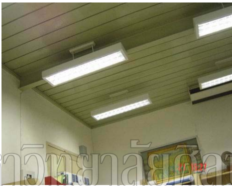
In the office ( Room no.1 ). Show metal I-beam at ceiling.
