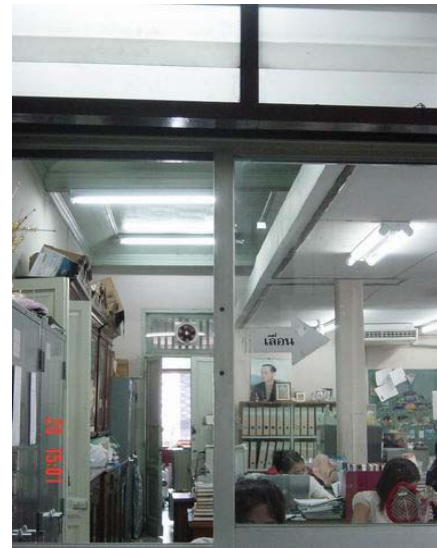
Inside the office room, the old column and beam of the terrace show in the room.
