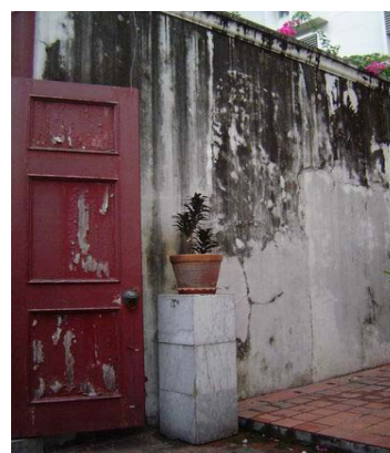
The only one left red old door and the residential area wall, view from inner court to the front of palace. Condition of wall is bad. Its materials are full of cracks and gigantic fungus stains. Condition of wood frames and panels of the old door is quite good except for color scratches and patches.
