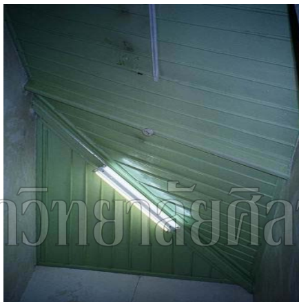
Angled ceiling seen from east to west.
