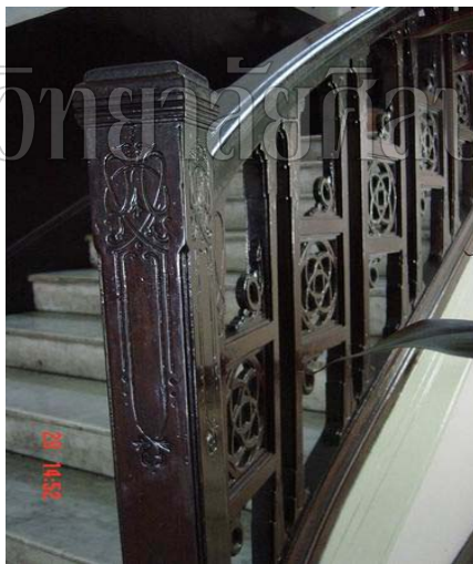
Detail of stair rail, sweet pattern of wood engraved and fretwork
