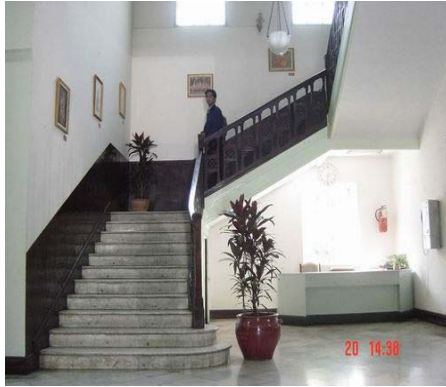
Staircase view from ground floor. White-gray marble floor, curved wood rail and brown color painted wall ( the same high as rail).
