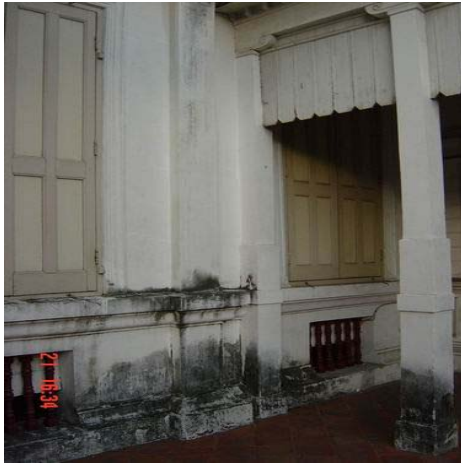
Picture of front elevation of the building.
