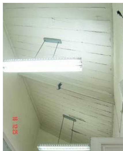
Figure 115 Office room in the front part of building. Its condition is old, having stains of damp, color peeling. Wood board ceiling crack.
