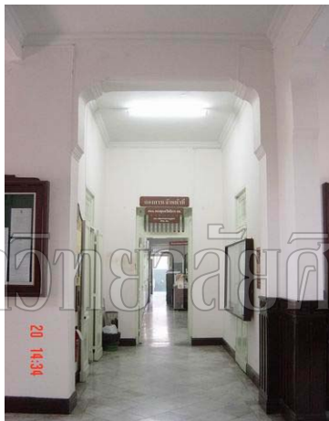
Corridor to north wing, far end has a door opened to outside
