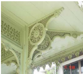
Pretty wood fretwork bracket under the roof of the pavillion.
