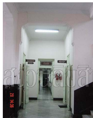
Corridor to south wing, far end is an office of one of deputy director
