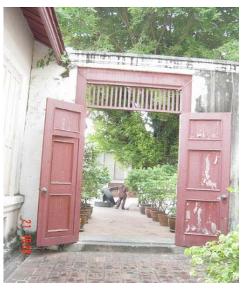
The only one left red old door and the residential area wall, view from inner court to the front of palace. Condition of wall is bad. Its materials are full of cracks and gigantic fungus stains. Condition of wood frames and panels of the old door is quite good except for color scratches and patches.
