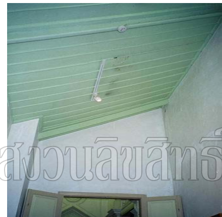
Angled ceiling over a connecting door to stair hall.
