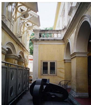
Space between building, view from north to south. It looks like the gallery intends to use this area for exhibiting arts object, but it should have information signs and inspired atmosphere.
