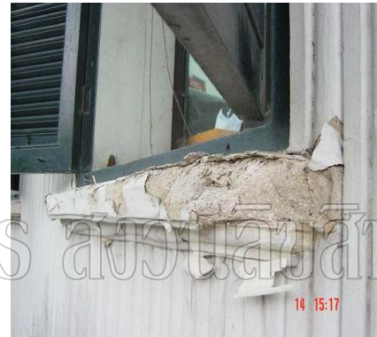
View of front elevation. Damage of wall and window-sill, Window-sills in the pictures seriously damaged, its color scratched and peeled to show lime mortar inside.
