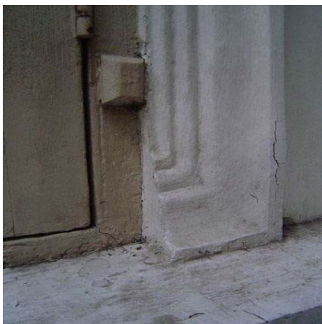
Figure 40 Wooden window and plaster architrave.
