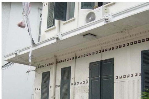
South elevation of the building, lower part wall has bad condition. Cement stucco cracks and exposes. Some parts of plaster decoration lost and has salt powder. Beneath the sunshade has bad condition too. Wall around the end of main pile decay.
