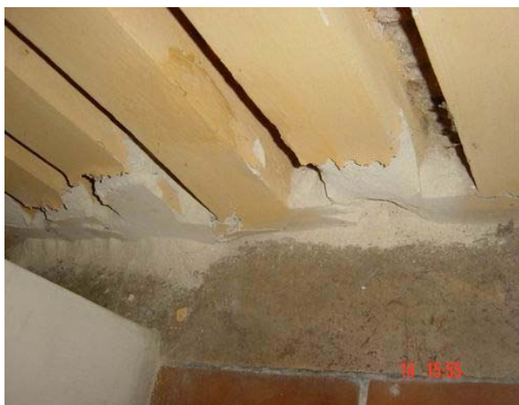
Lime wall explosion and having efflorescence effect
