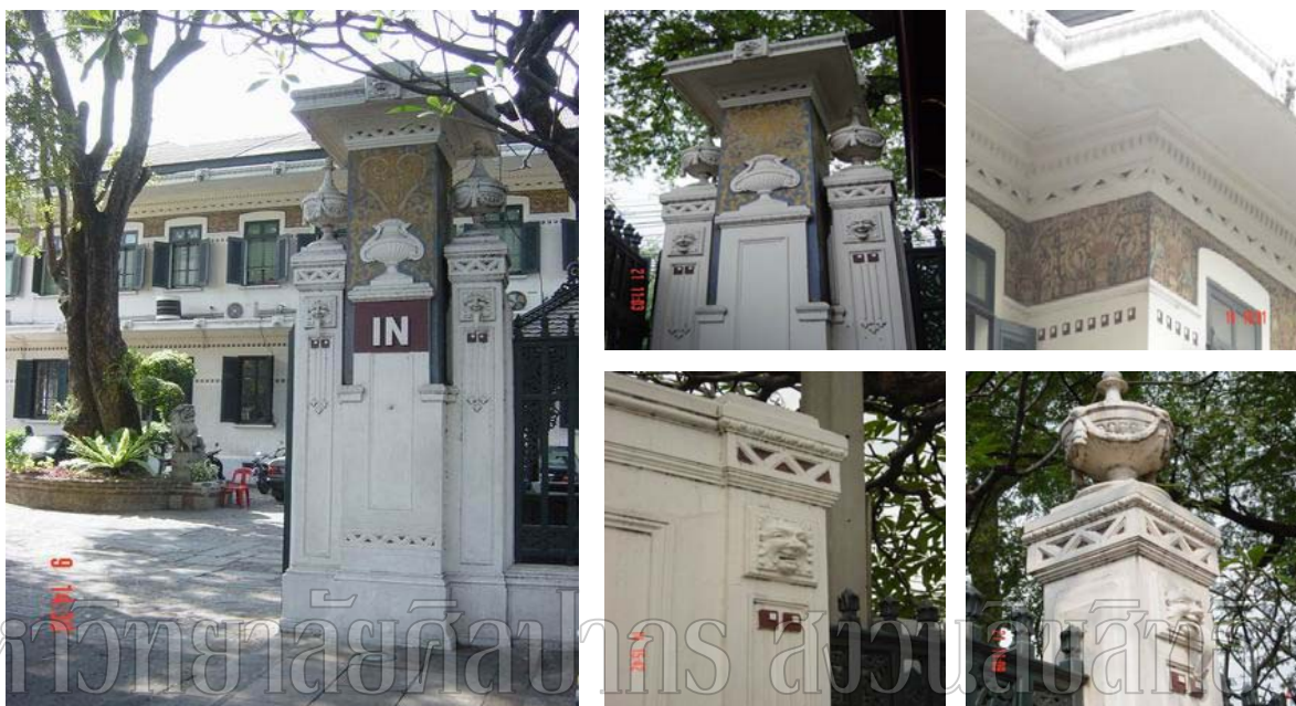
Figure 121 Beautiful and unity design of the office building and fence.
