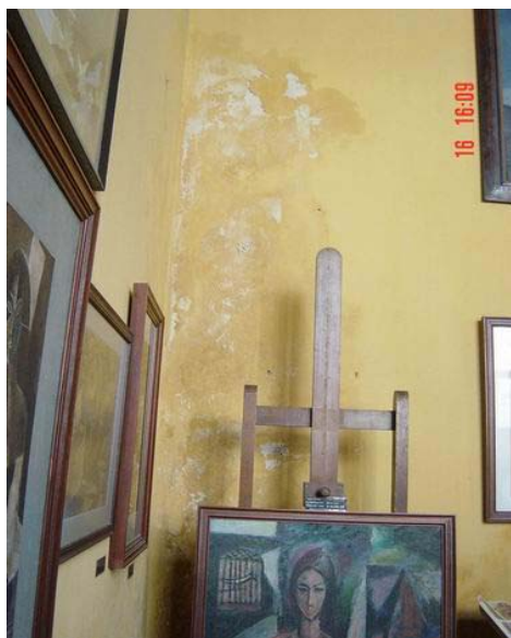
Wall painting is scratching and peeling. The serious problem is lime stucco corrosion.
