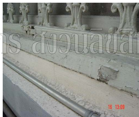
Figure 108 Beautiful metal curved railing is in a good condition but wall plaster moulding and wooden frames of window are in bad damage of color peeling and scratch.
