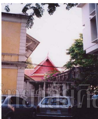
View of west elevation; A disturbing vision of the heritage place, disorder electrical wires, dirty stains on fabric of buildings, for instance.
