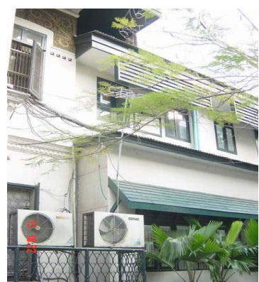
Back of the building, north wing, views inside Silpakorn university. This north wing close to the building of Faculty of Fine Arts, Sculpture and Printing
