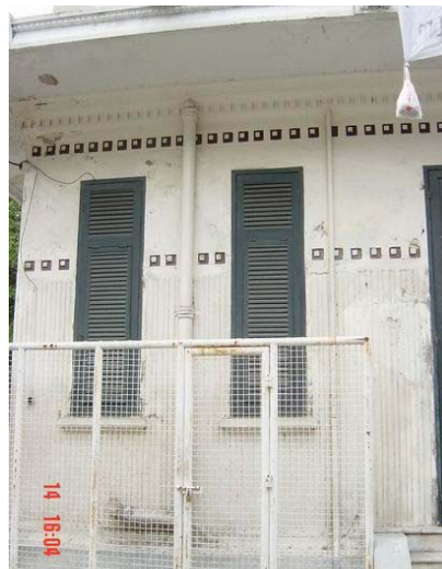
South elevation of the building, lower part wall has bad condition. Cement stucco cracks and exposes. Some parts of plaster decoration lost and has salt powder. Beneath the sunshade has bad condition too. Wall around the end of main pile decay.
