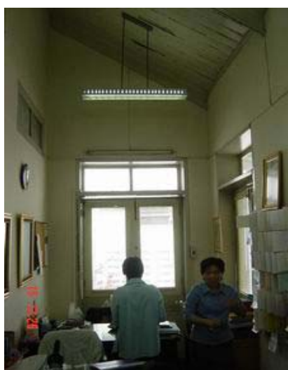
Figure 115 Office room in the front part of building. Its condition is old, having stains of damp, color peeling. Wood board ceiling crack.
