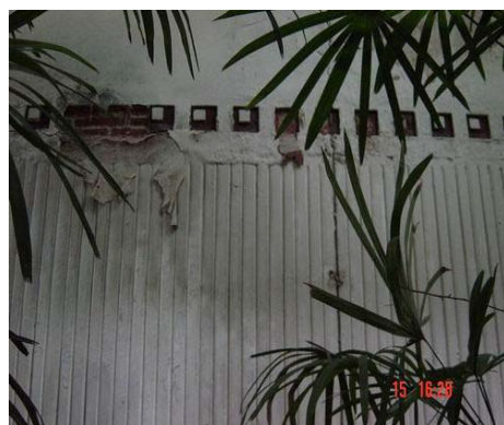
Back of the building show serious damages of wall and sunshade. Some significant decoration lost.
