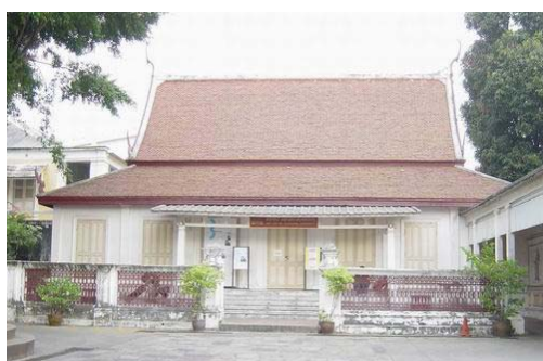
Thong Phra Rong view from the front. Although less elaborated, Thong Phra Rong has fully elegance of Thai style architecture.
