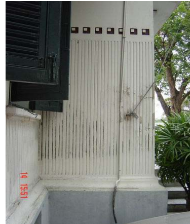
Many parts of the front wall discolor and stain with fungus and wet water. Color painted scratches and peels.
