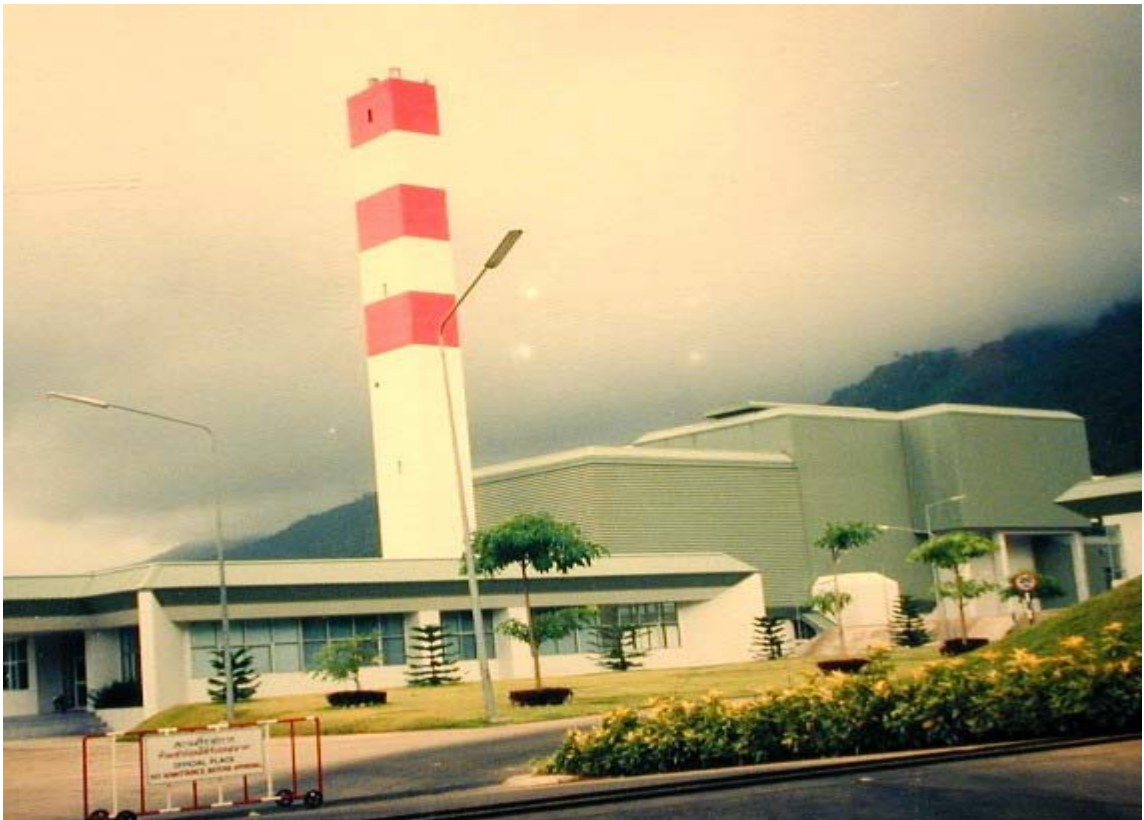
Figure 4-7 : Samui Solid Waste Incineration Plant.
